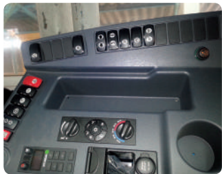
Centralized Instrument Switch Panel
